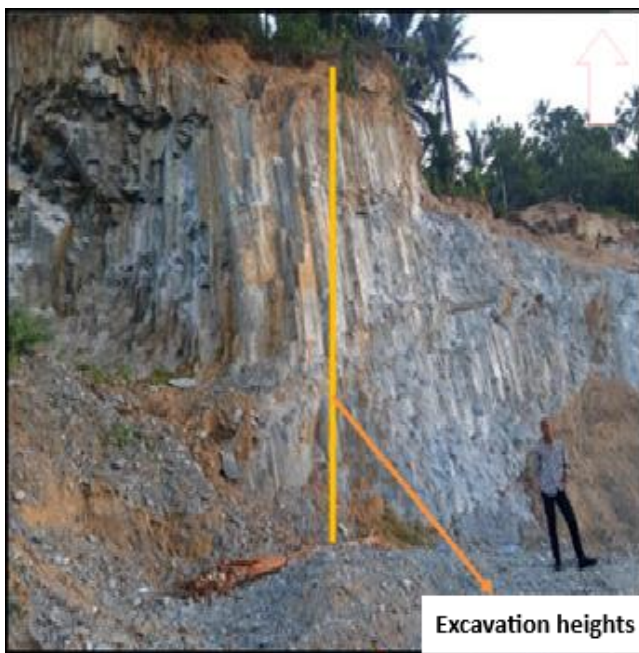
Figure 6. Documentation Excavation wall height
